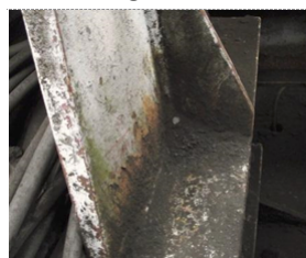
Fig. 2. Welded corner joint in T shape
